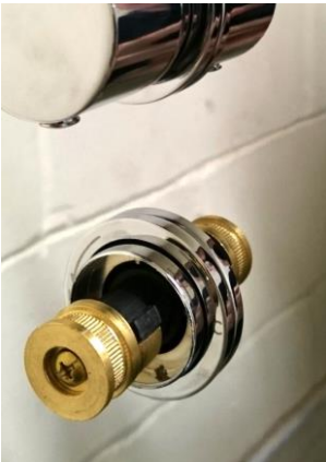
3. The Temperature Handle Bush is now visible.
